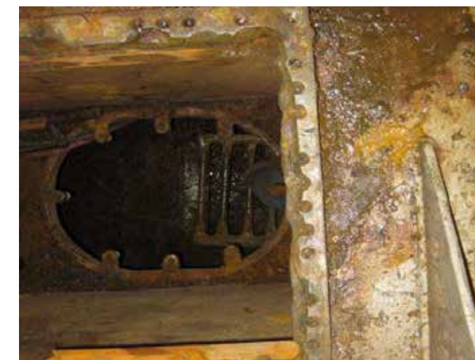
Above: An example of box-cooler compartment corrosion from The Club's archives
